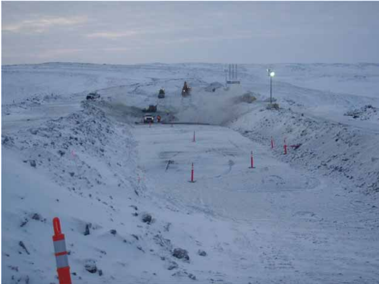
Photo 1: ~W view down key trench towards the start of dayshift FCM placement.
