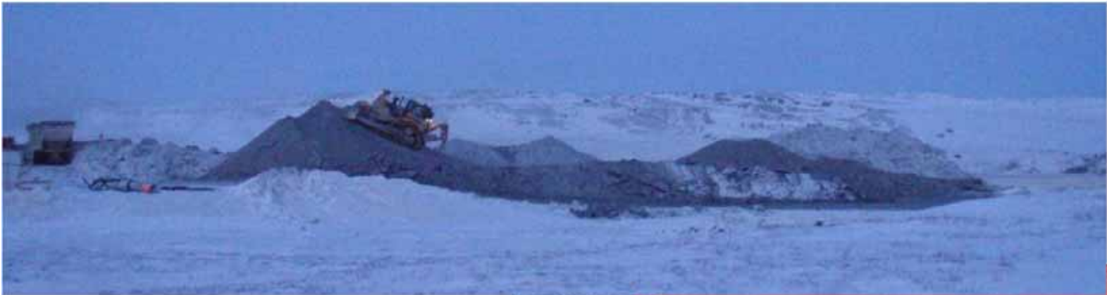
Photo 2 (top middle): ~ E view of D9 working on breaking up frozen lumps at the FCM stockpile on the FCP Pad
