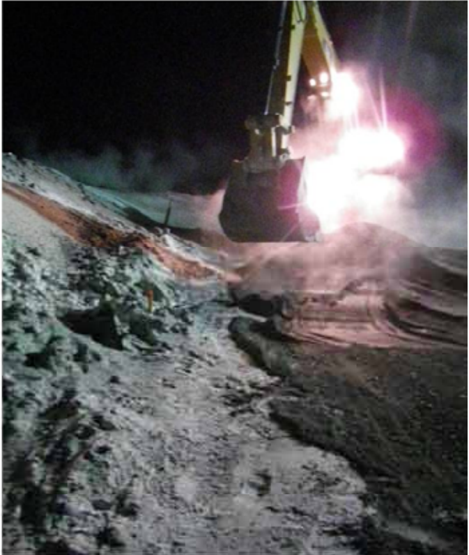
Photo 15: Excavator placing FCM along the upstream edge of the key trench near station 0+60.
