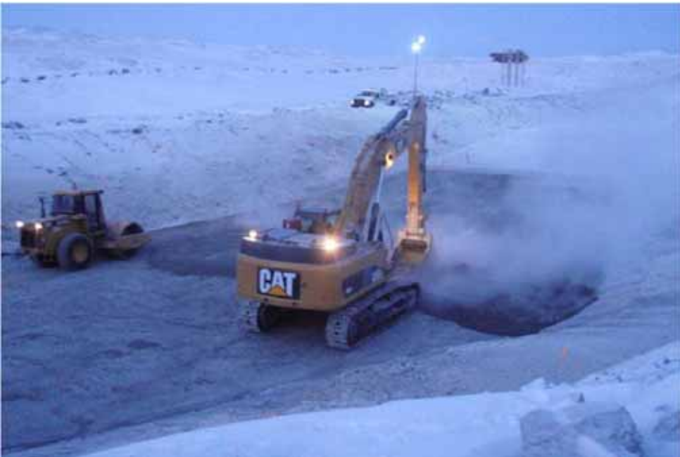
Photo 4: ~NNE view of the 345 excavator spreading FCM around station 0+90.
