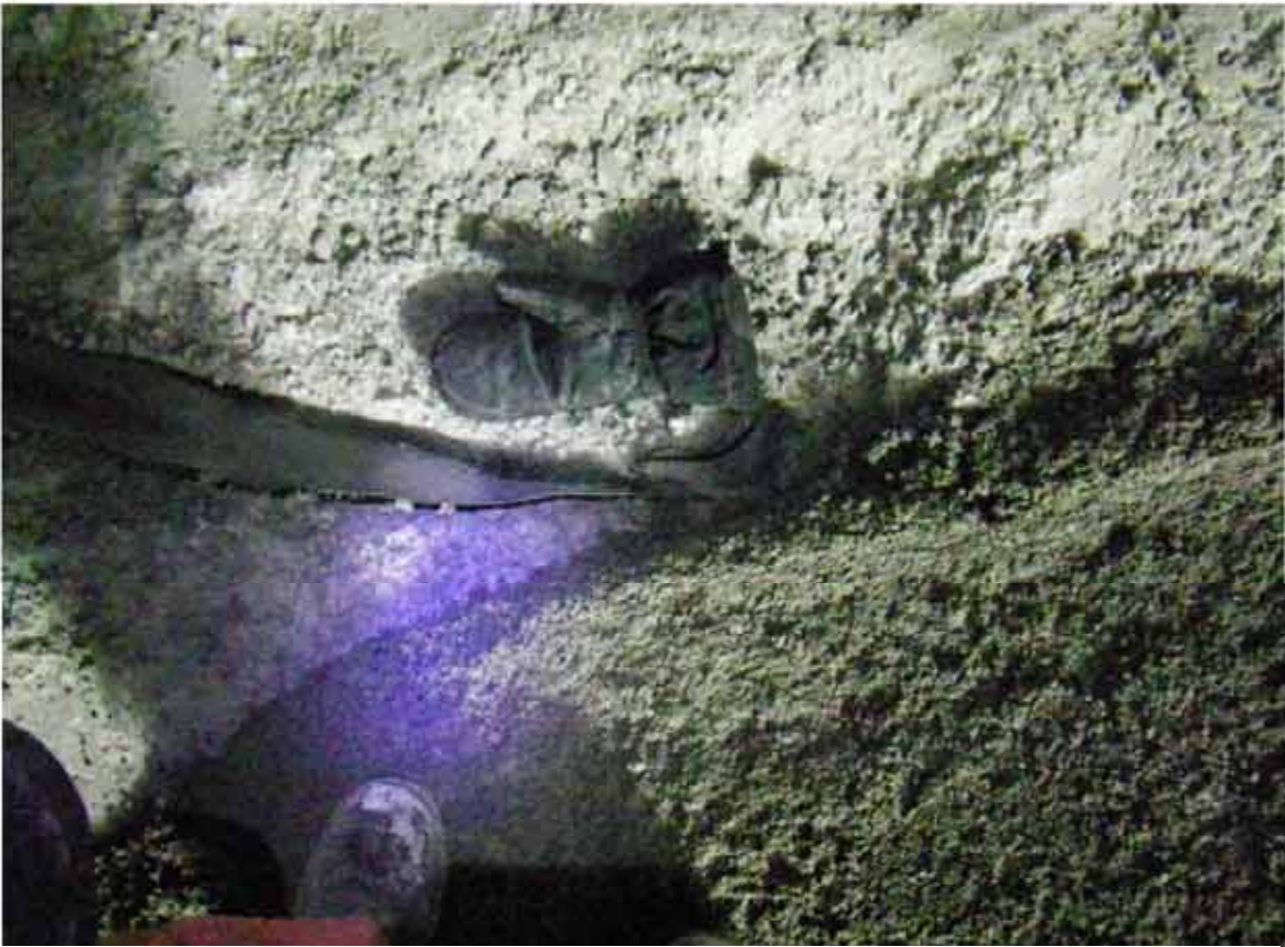
Photo 16: FCM placed on the upstream slope very close to possibly on the HDPE liner which is protecting the GCL. The HDPE will have to be removed and the GCL in the coming days.
