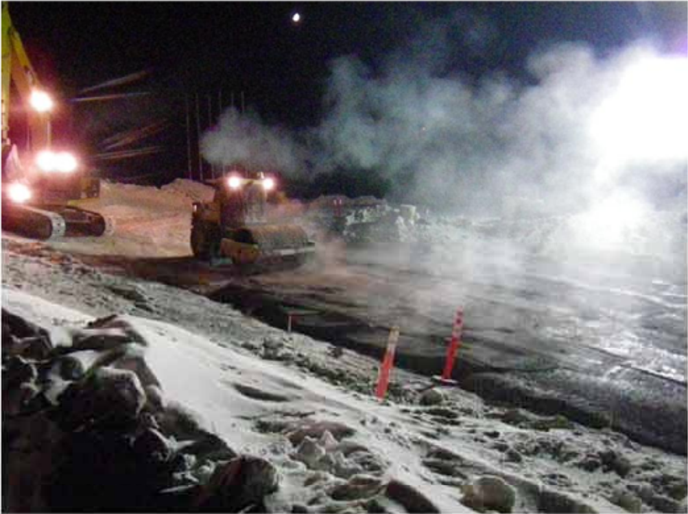
Photo 14: Compactor running on material placed during the night shift.
