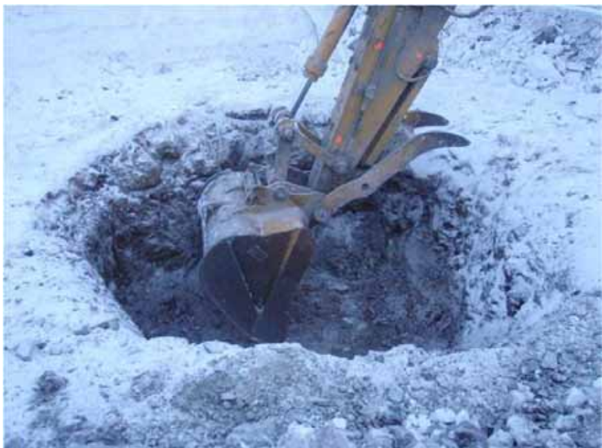
Photo 5: View of 325 excavator boom (with finishing bucket) working on the Sump #2 excavation.
